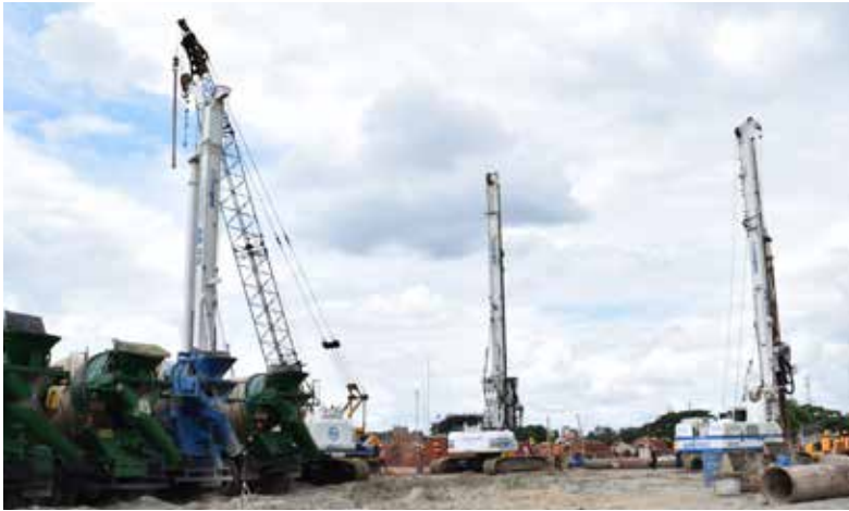
Construction of 600 Ø Depth- 30m, Nos- 254 bored RC pile for 450 MW combined cycle power plant (north), Ashugonj.
