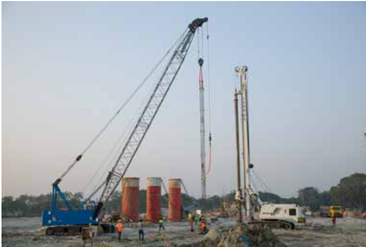
Rebar cage installation with the help of crane.
