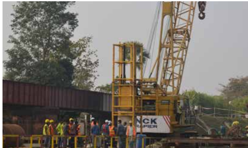
Dhaka-Chittagong Railway Development Project (DCRDP) Track doubling between Laksham and Chinki Astana, high strain dynamic testing of pile.
