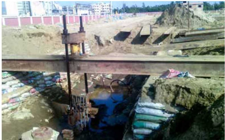
Uplift pile load test.
