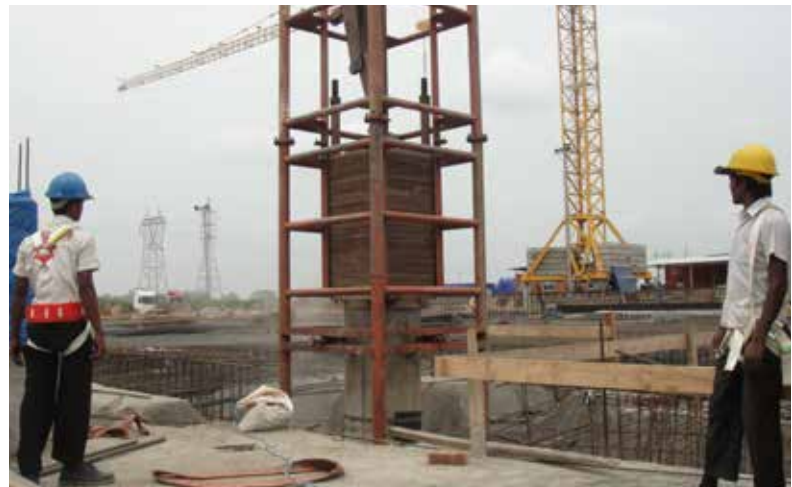
Saidabad water treatment plant phase-II Dhaka high strain dynamic testing of pile.
