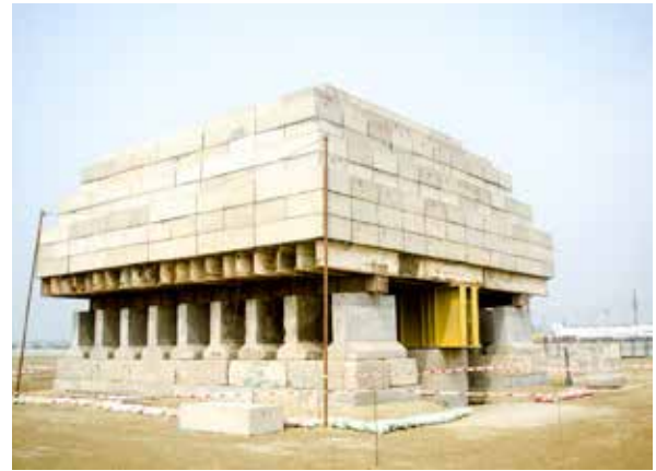
Dhaka Mass Rapid Transit Project CP-02 966 Ton pile load test.
