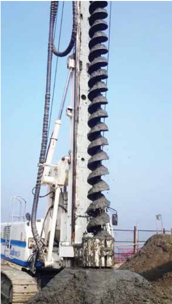
CFA Boring, Ashugonj Power Plant, Soilmec SR30.
