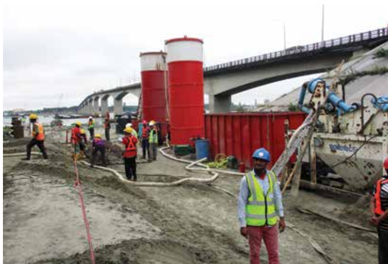
Construction of 600 \phi Depth- 24m, Nos- 121 bored RC pile for Meghna bridge under Kanchpur, Meghna, Gumti 2nd bridge Rehabilitation of existing bridge project.
