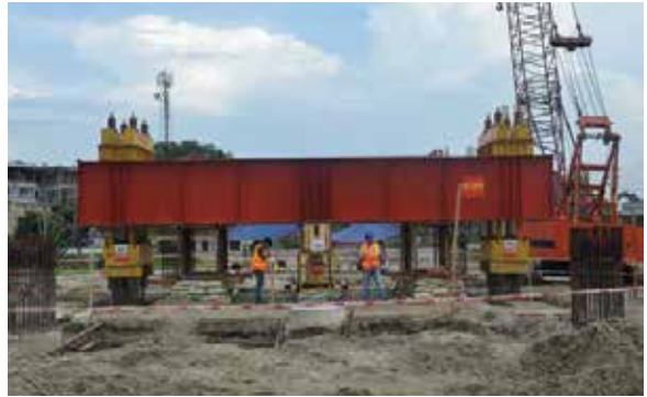
450 MW combined cycle power plant (south), Ashuganj 1250 ton pile load test.
