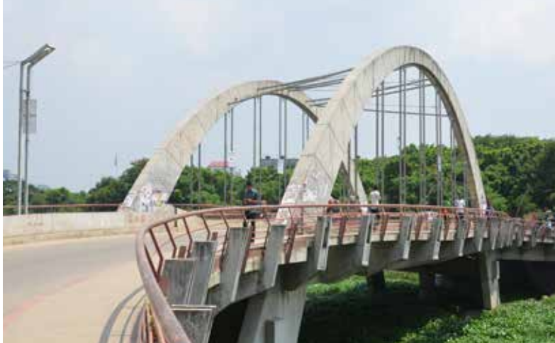
Construction of 900 Ø Depth-30m bored RC pile for Banani-Gulshan link bridge LGED on Banani-Gulshan road, Dhaka.
