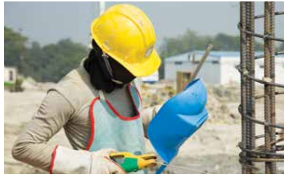
Rebar Cage Welding.
