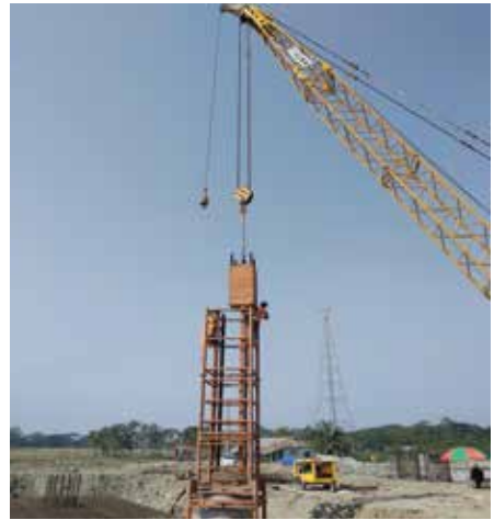
Payra Bridge project, Lebukhali, 900 MT PDA Test.
