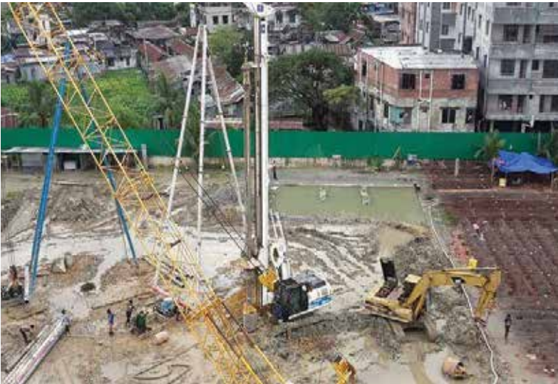
Construction of 1000 Ø Depth-48m, Nos- 331 bored RC pile for PGCB Head Office Building, Aftabnagar, Dhaka.
