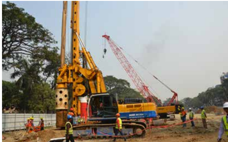
Construction of 1000 \phi , 1200 \emptyset , 1500 \phi & 2200 \phi Depth- 35m bored RC pile for DMRT Line-6, CP-05.
