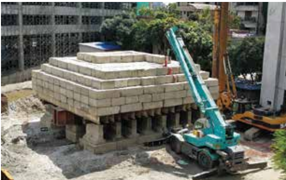
Pile Load test for Swissotel, Dhaka-900 MT.
