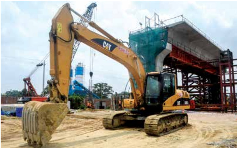
Excavator, Caterpillar 320C.
