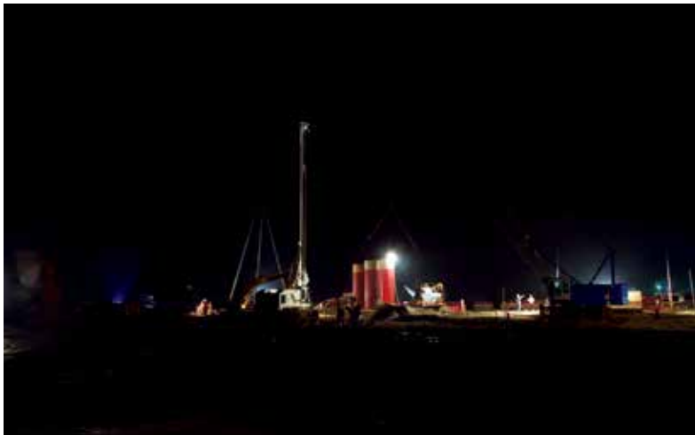
Construction of 600 Ø Depth- 28m, Nos- 154 bored RC pile for British American Tobacco, Kushtia.
