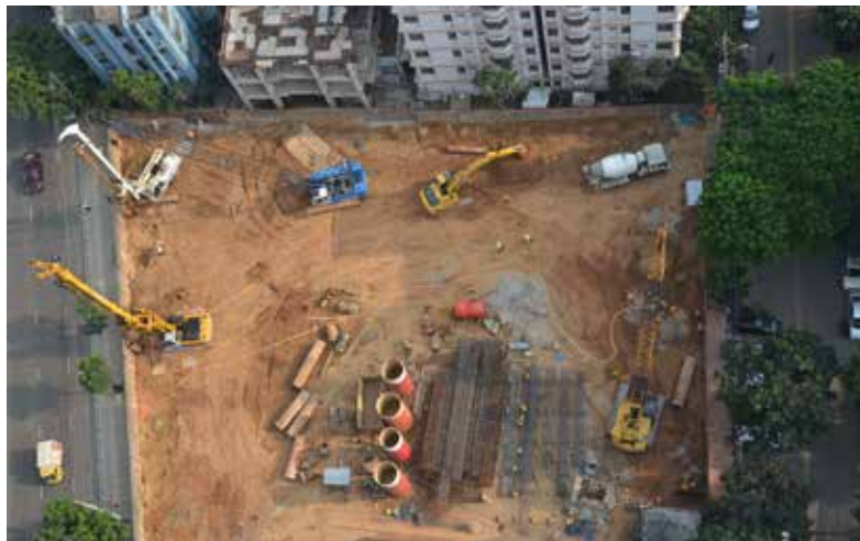
Construction of 600 \phi , 1000 \phi & 1200m \phi Depth- 28m, 37m, 52m, Nos- 305 bored RC pile for South Park (Westin Hotel, Dhaka), Gulshan, Dhaka.
