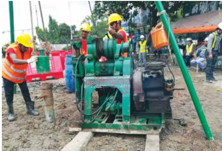
Rotary boring rig YBM-2.
