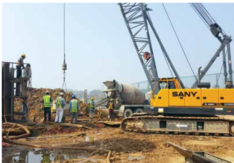
Construction of 1000 \phi Depth- 44m, Nos- 408 bored RC pile for First Elevated Expressway, Dhaka.
