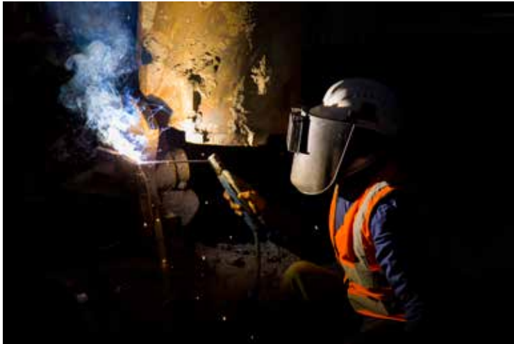
Drilling tool repairing.
