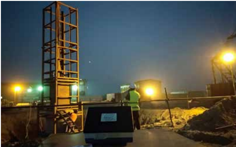
Khulna-Mongla Railway Project, Rupsha Bridge high strain dynamic testing of pile.
