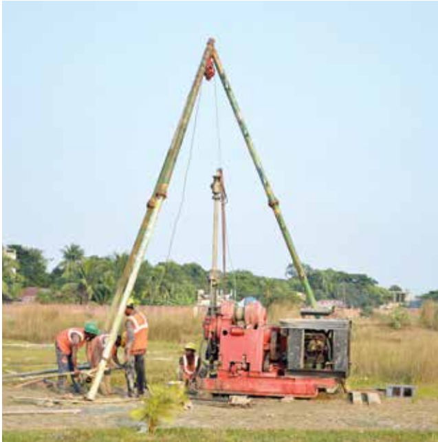
Spindle type rotary boring rig, Tone boring TBM-188.
