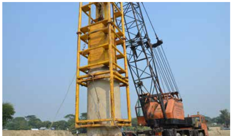
Janjira approach road & selected bridge facilities ICB: PMB/01 high strain dynamic testing work of pile.
