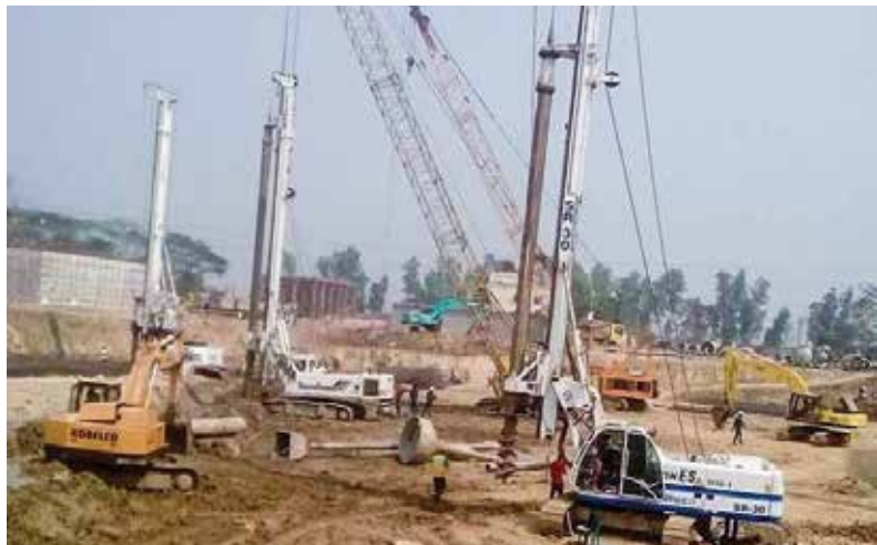
Construction of 600 \phi Depth- 24m, Nos- 1085 bored RC pile for 275 MW Coal fired power plant at Barapukuria, Dinajpur.
