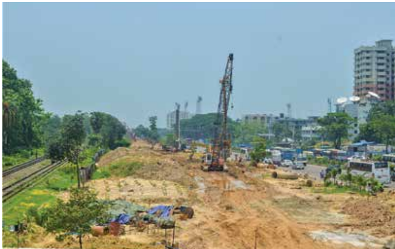
Construction of 1000 Ø & 800 Ø Depth- 44m, Nos- 408 bored RC pile for First Dhaka Elevated Expressway.
