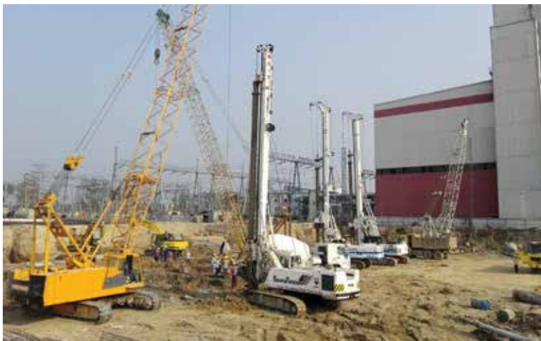
Construction of 600 Ø Depth- 24m, Nos- 1085 bored RC pile for 275 MW Coal Fired Power Plant Barapukuria.
