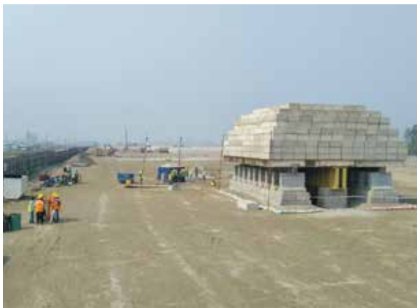
9625kN Static Load Test, Dhaka Mass Rapid Transit (DMRT) Project, Line 06, CP-02.
