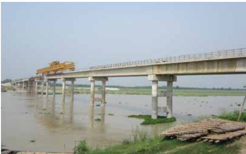
Construction of 1000 Ø Depth- 45m bored RC pile for Mohanondha Bridge, Chapai Nawabgonj.
