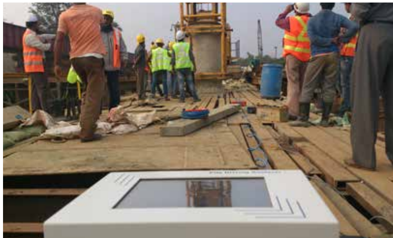
Sayed Nazrul Islam Medical College, Kishoregonj high strain dynamic testing of pile work.
