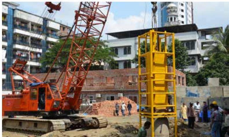
Moghbazar-Mouchak Flyover 1500 MT PDA Test.
