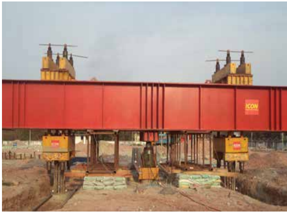
Dhaka-Chittagong Railway development project (DCROP) Track doubling between Laksham-Chinki Astana 700 ton pile load test.
