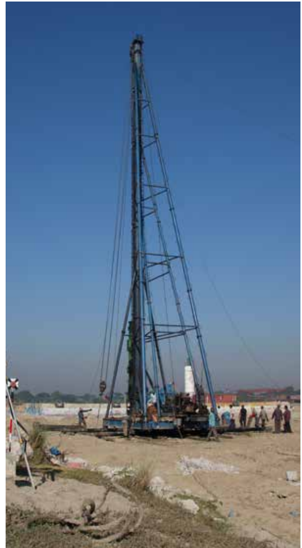
Skid Mounted pile driver.
