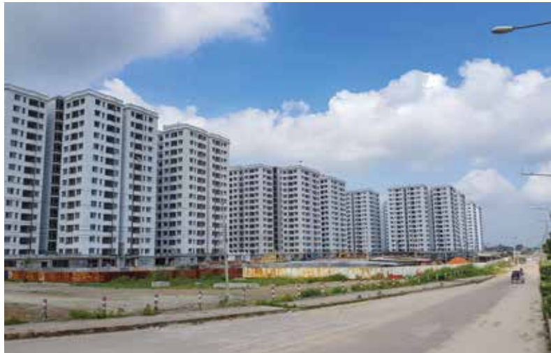
Uttara Apartment of RAJUK on 400 Square Concrete Driven pile.
