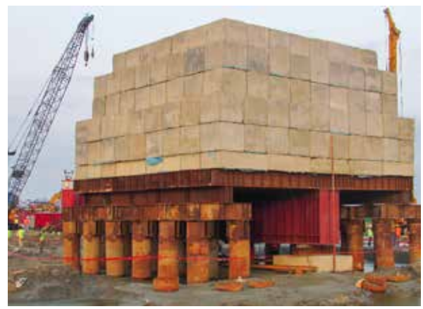
Khulna-Mongla Railway Project Larsen & Toubro 1350 ton pile load test.
