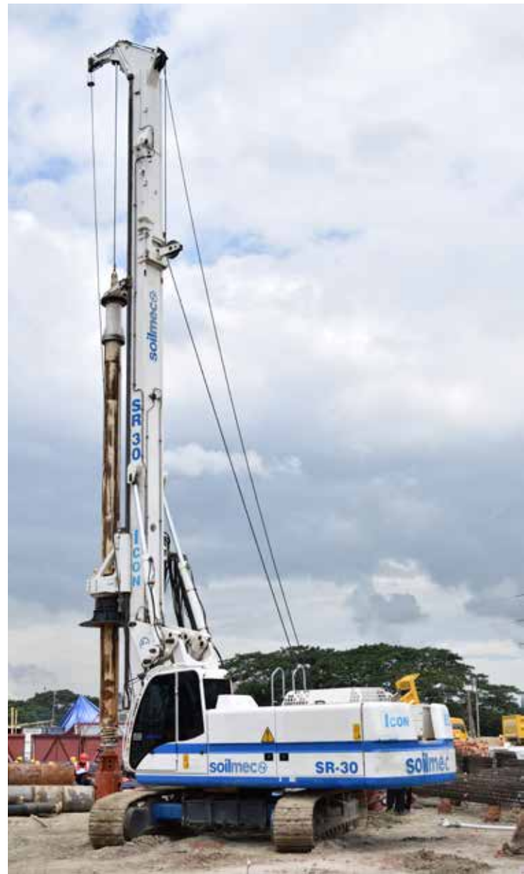
Soilmec SR-30, Italy.
