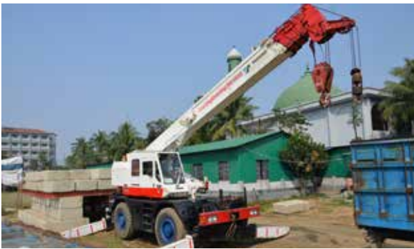
Rough Terrain Crane.
