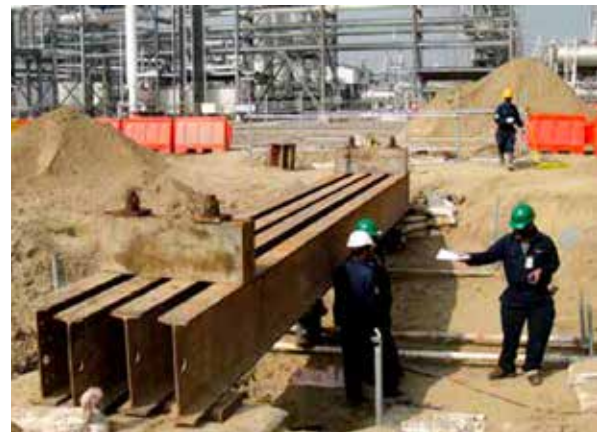
Bibiyana Expansion Project Vertical pile Load test.
