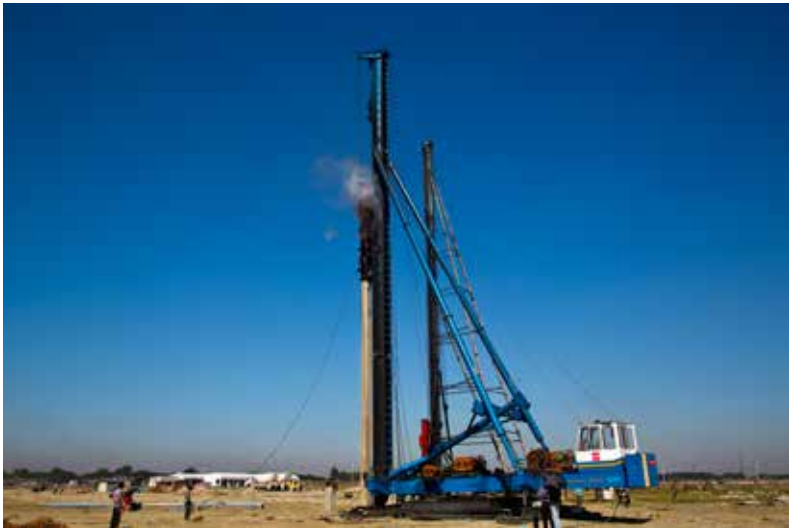
Uttara Apartment Project, Dhaka 400mm square, 35m long, Nos-3800 pre-cast pile, D46 diesel hammer in operation.
