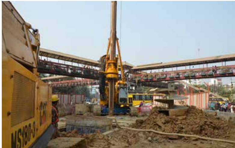
Construction of 1800 \phi bored pile for DMRT Line-6, Cp-04, Mirpur-10.
