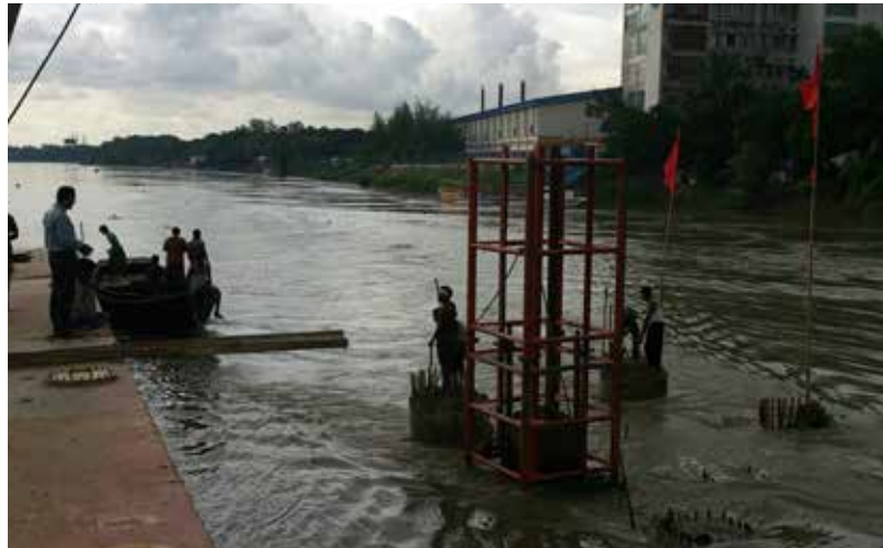
Bridge over Shikolbaha River, Chittagong high strain dynamic testing of pile.
